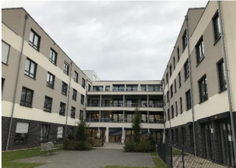
Combined nursing home and assisted-living facility – Papenburg, Lower Saxony, Germany
